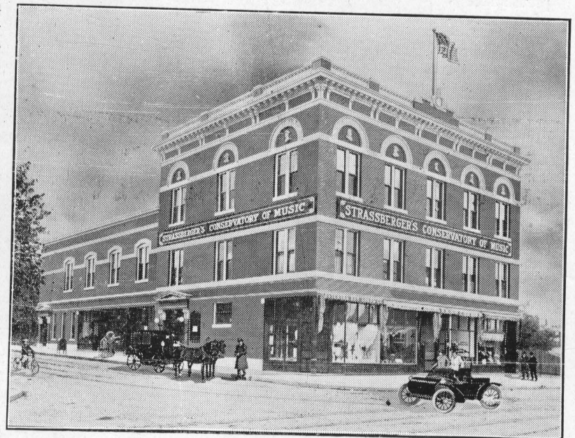
SOUTHSIDE CONSERVATORY BUILDING
